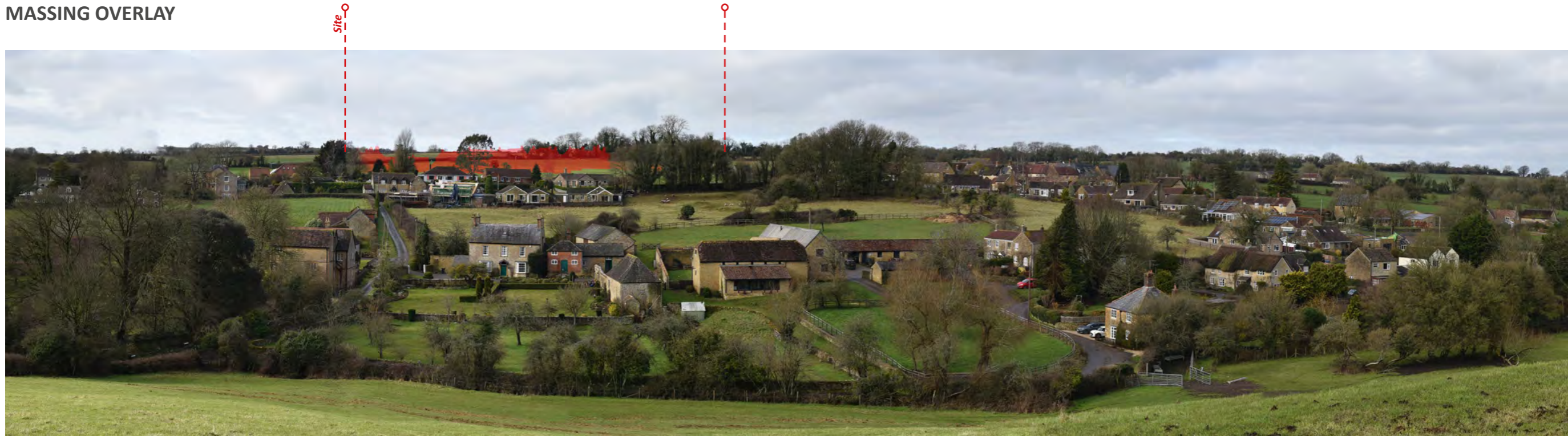
VIEWPOINT 1: Illustrative view from PRoW looking west towards the Site with proposed massing.
